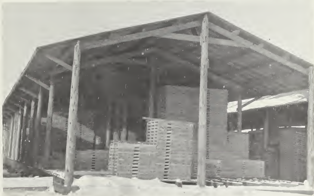
Figure 39. --An air-drying shed of the pole-barn type.
